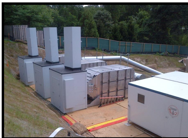
Sound suppression structures designed and built by the team to allow the noisy CAFS filters to run quietly overnight in the residential neighborhood.
